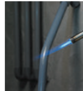
PVC pipes work.
